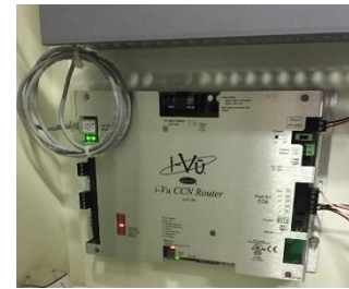
Image 8: HVAC Control System
