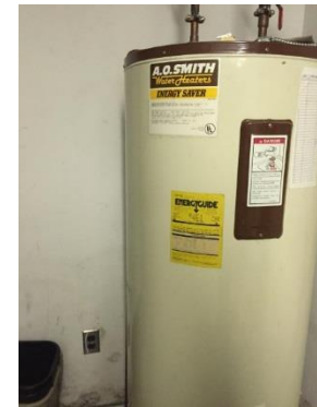
Image 9: Domestic Hot Water Heater
