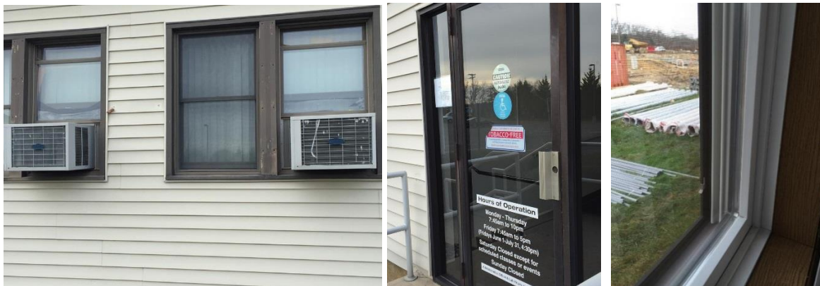
Image 1: Building Exterior, Windows, and Doors
