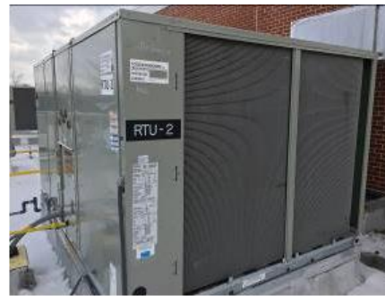
Image 8 – Roof Top Unit #2 (Serves Gym)
