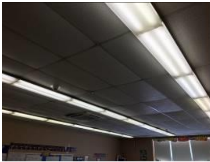
Image 3 – T8 Fluorescent Lighting
