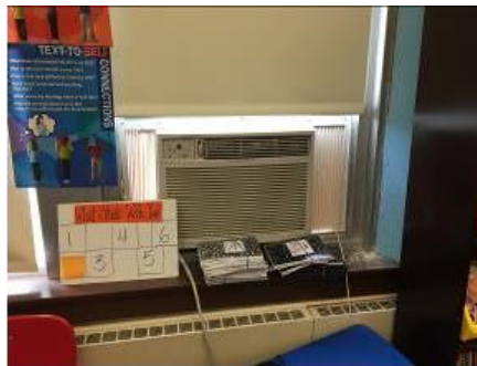
Image 7 – Window AC and baseboard (Office)
