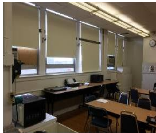
Image 4 – T8 Fluorescent Lighting
