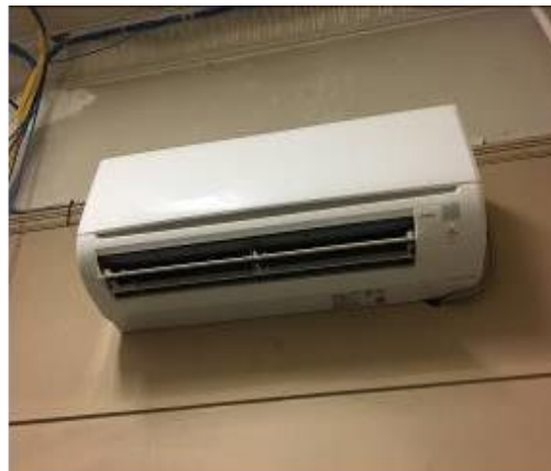
Image 8 – Split HP Indoor Coil Unit (Server Room)
