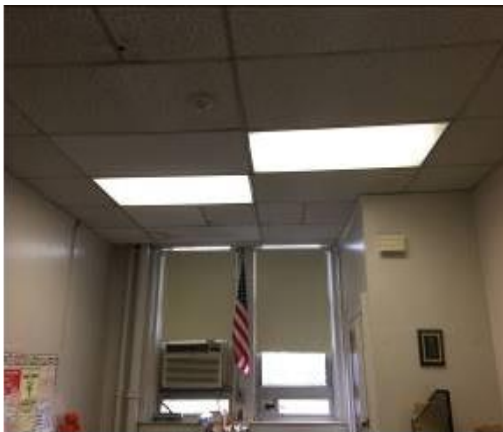
Image 3 – T8 Fluorescent Lighting
