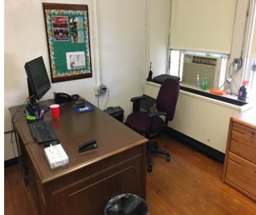
Image 7 – Window AC (Offices)
