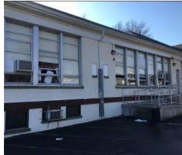
Image 8 – Window AC (outside view)
