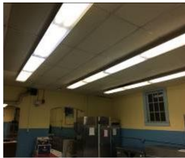
Image 3 – T8 Fluorescent Lighting
