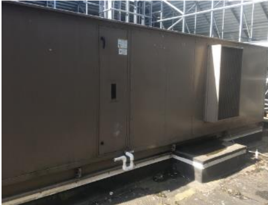
Sample Air Handler
