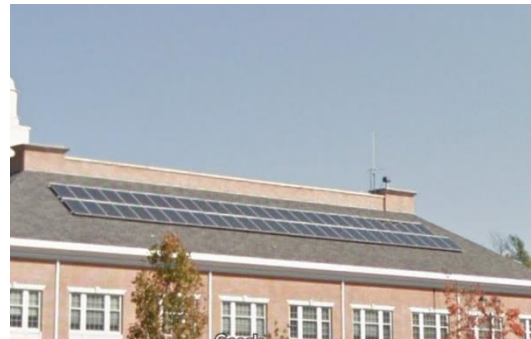
Facility South Side
