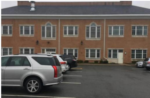
Facility North Side
