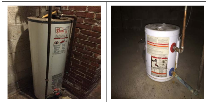
Image 8: Domestic Water Heating System
