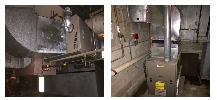
Image 6: Gas Fired Furnaces
