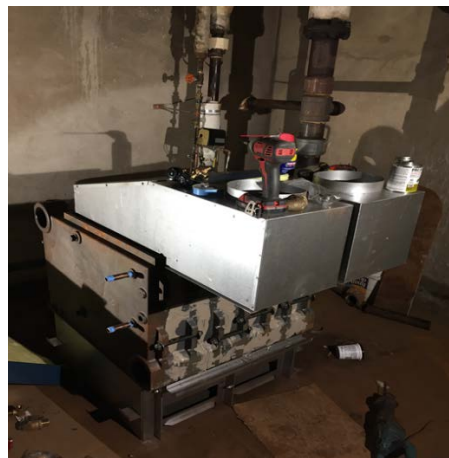
Image 4: New Boiler Under Installation
