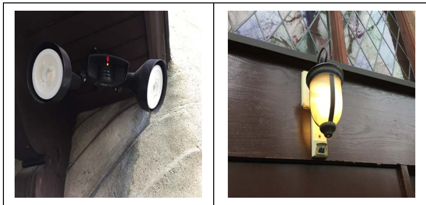
Image 3: Exterior LED & HPS Fixtures
