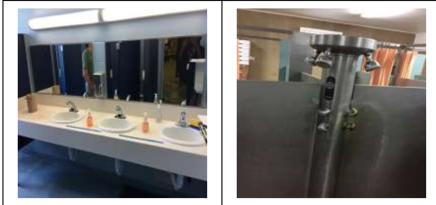
Image 8: Typical Restroom & Shower Room Faucets
