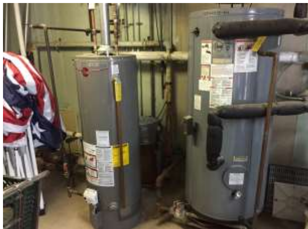
Image 7: Domestic Water Heaters
