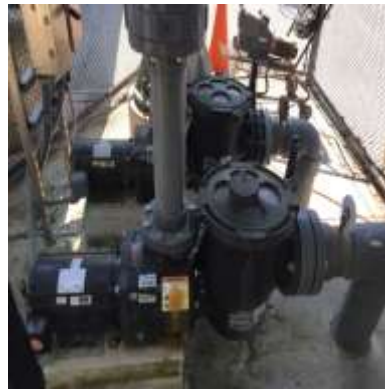
Image 6: 15 hp Water Slides Water Supply Pumps
