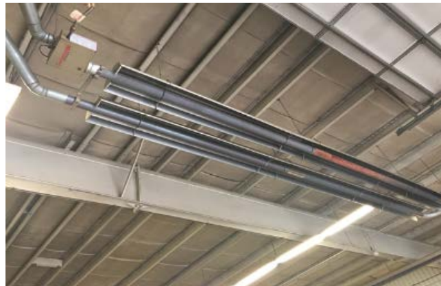
Image 4: Garage Warm Air Unit Heater
