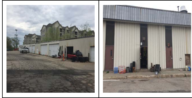
Image 1: Supplies and Main Building Envelope
