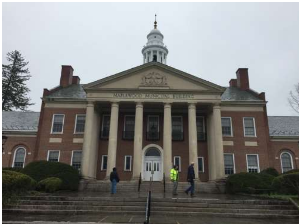
Image 2: Town Hall Building Envelope
