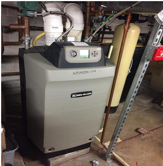
Image 4: Condensing Boiler
