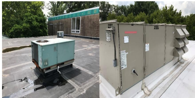
Image 5 Packaged AC and HV Unit
