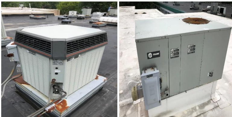
Image 4 Roof top units
