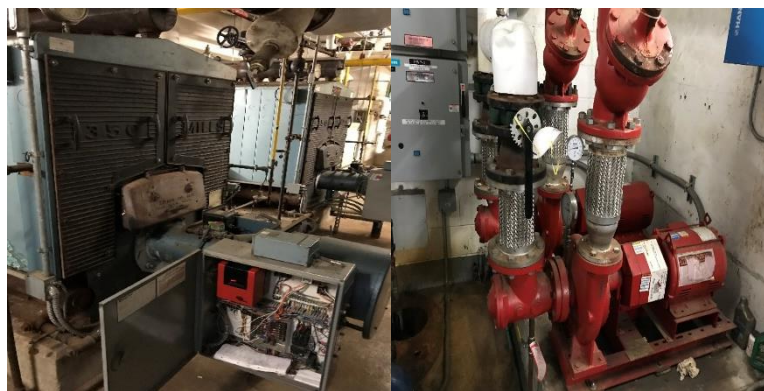
Image 3 School Boiler plant & heating pumps
