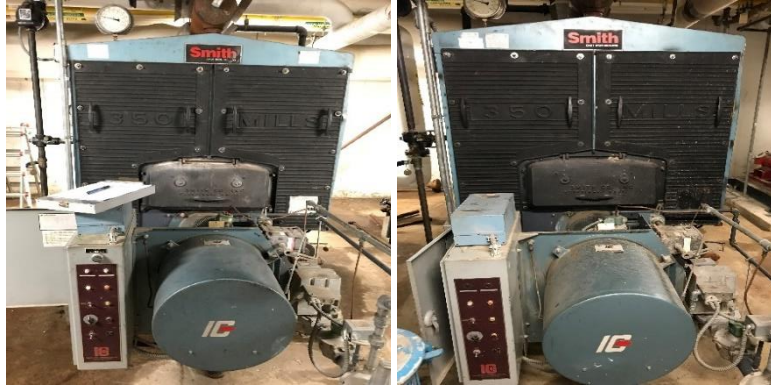
Image 4 School Boiler System
