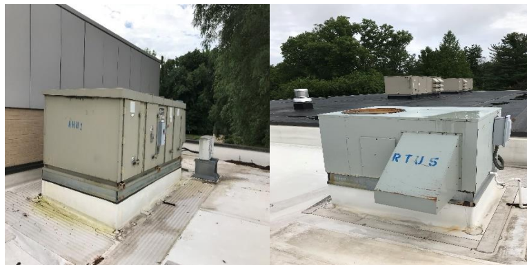
Image 5 AHU & Roof Top Unit
