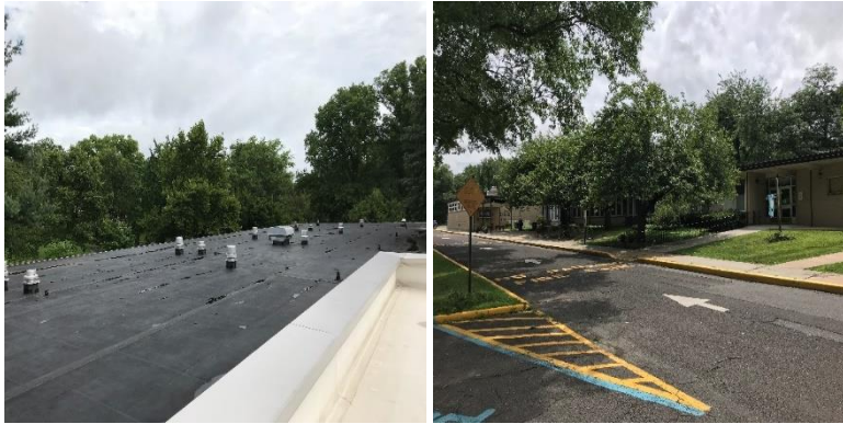
Image 1 Building Roof and Exterior
