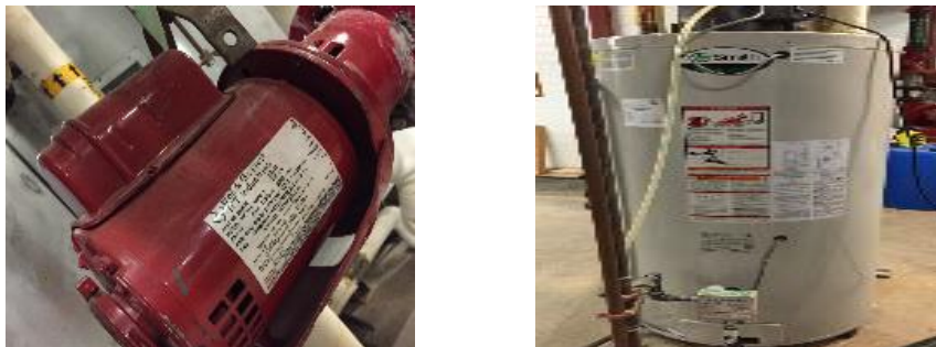
Figure 12 – Domestic Hot Water System
