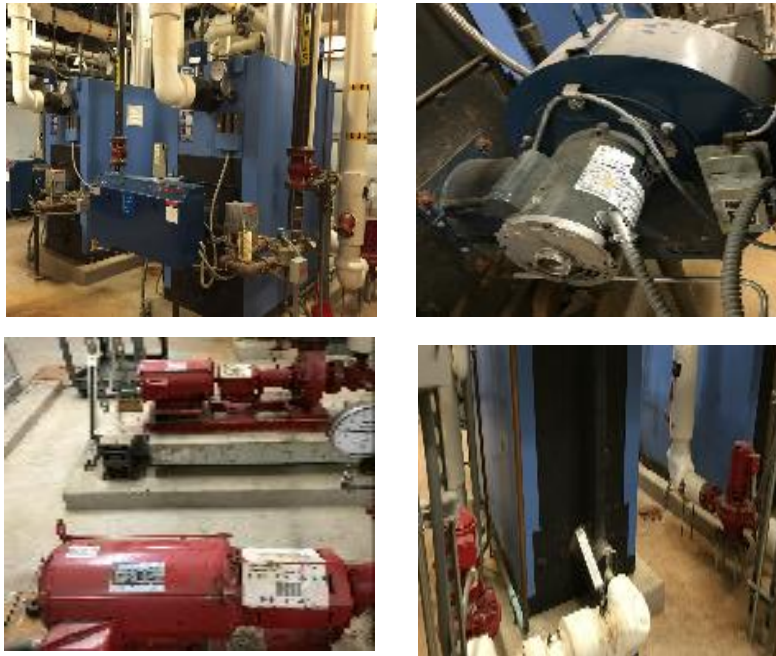
Figure 10 - Building Hot Water Heating System
