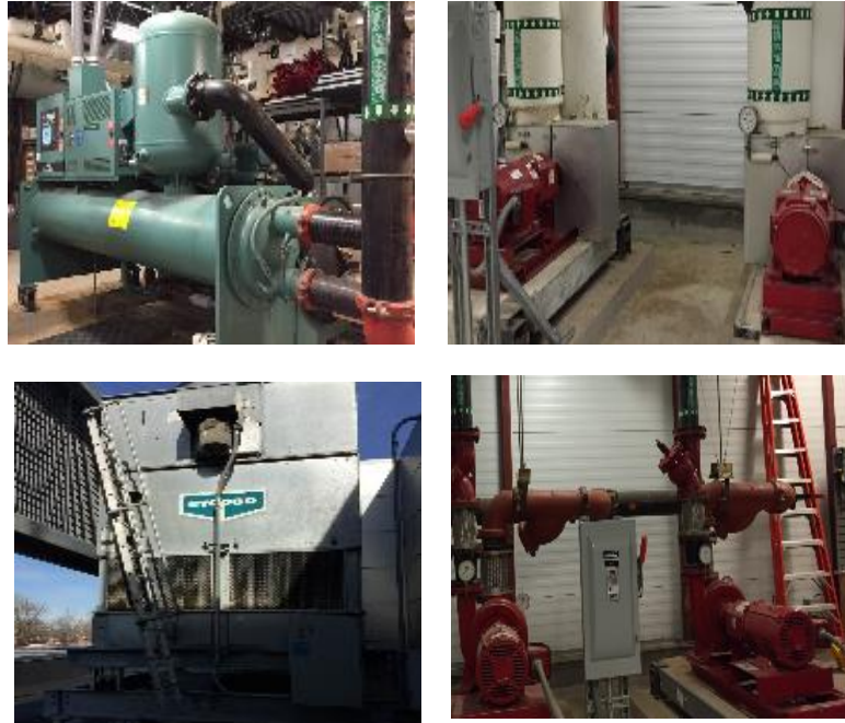
Figure 9 - Building Chilled Water System
