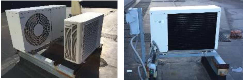
Figure 11 - Building Air-Conditioning Split-Systems
