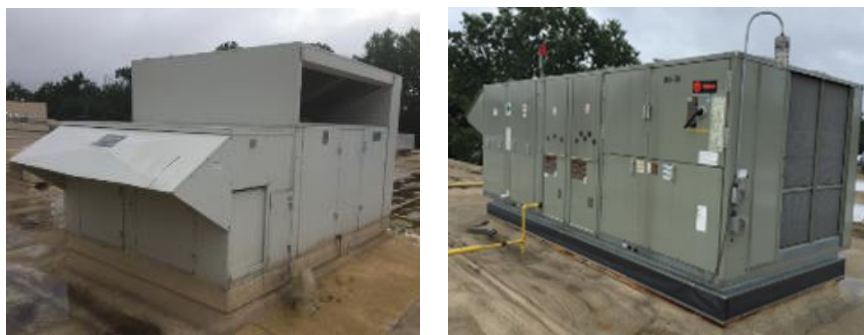
Image 10: Roof Top Package Units
