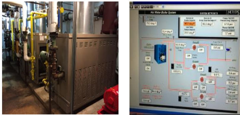
Image 8: Non-Condensing Hot Water Boilers
