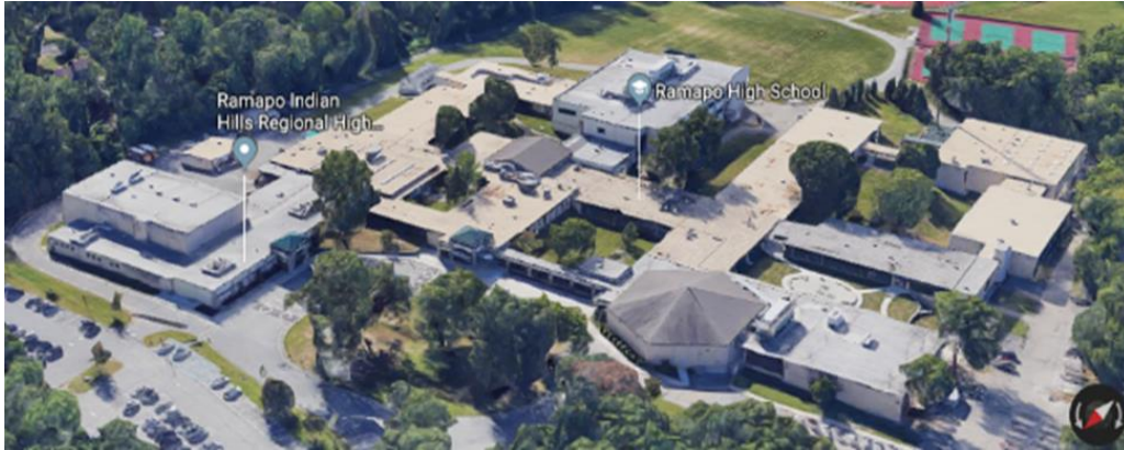
Image 2: Facility Aerial View
