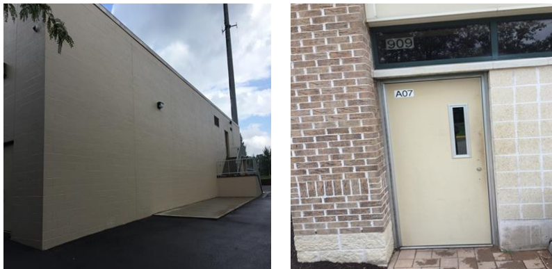
Image 3: Typical Walls & Exterior Door
