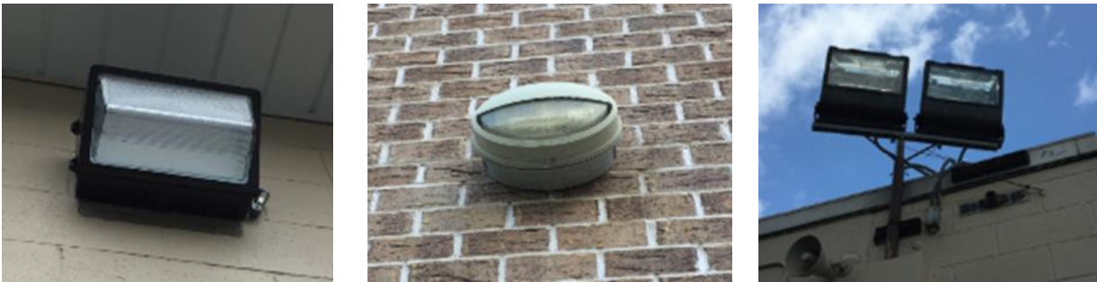
Image 7: Typical Exterior Wall pack Fixtures
