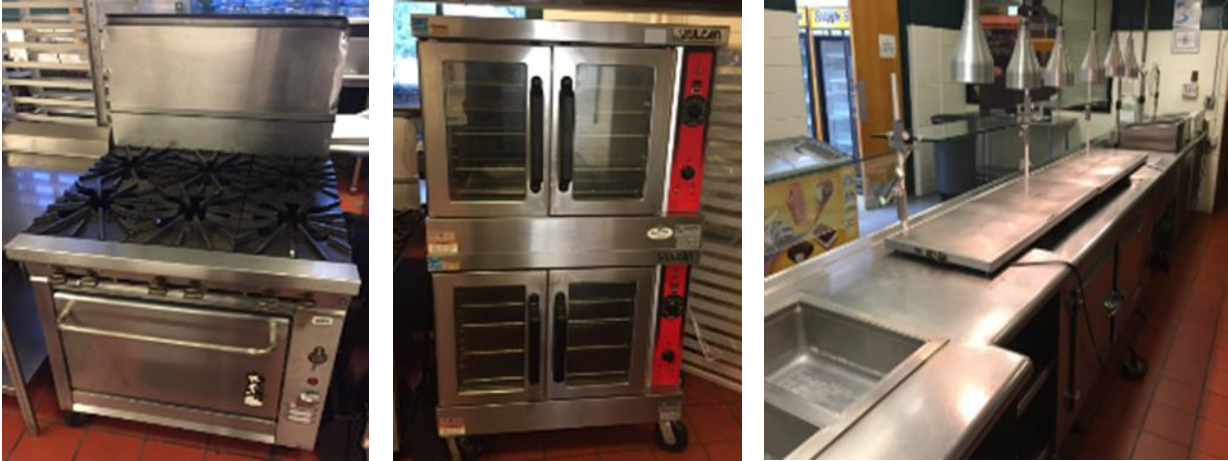
Image 13: Kitchen Gas Cooking Equipment & Steamers
