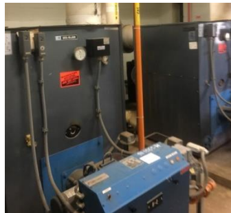
Advanced Treatment Boilers
