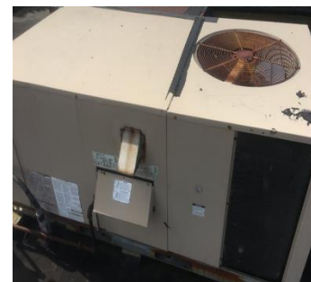
Lab Building Packaged AC
