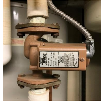
Image 22 Taco recirculation pump
