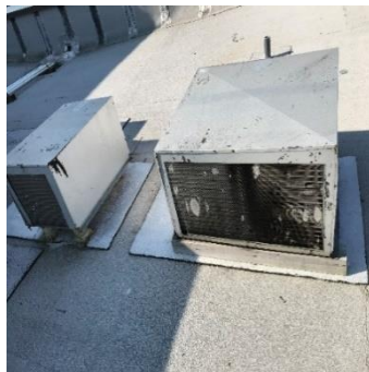
Image 29 Condensing unit on roof
