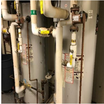
Image 21 Two hot water heaters
