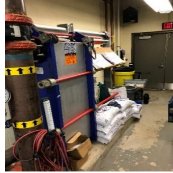
Image 14 Heat exchanger
