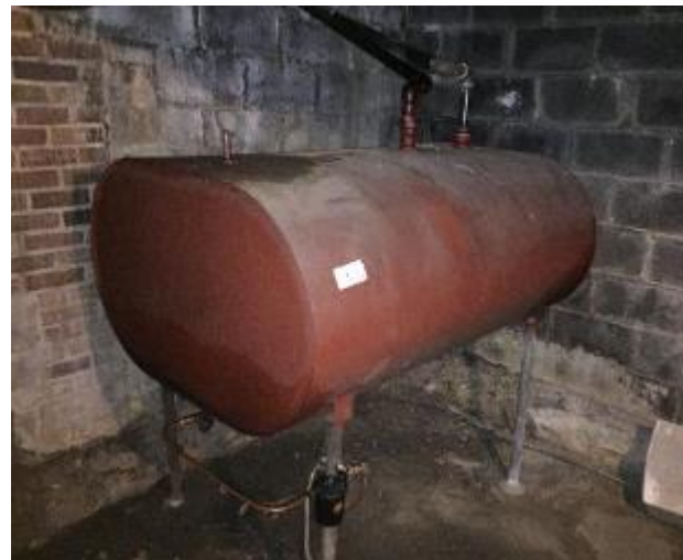
Image 5: Boiler Oil Tank
