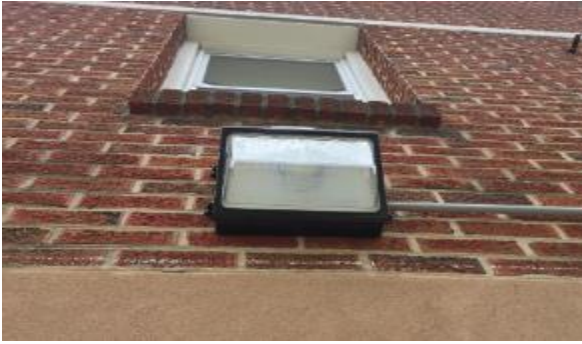
Image 2: Exterior Metal Halide
