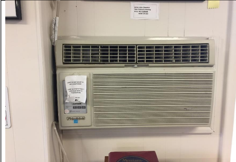
Image 5: Window AC (Inside)
