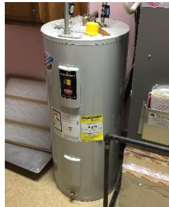
Image 4 Domestic Hot Water Heating System
