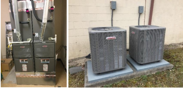
Image 3 Heating and Air Conditioning System
