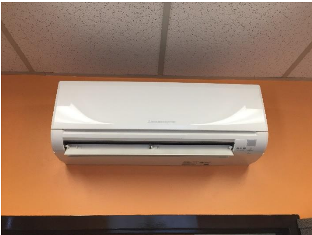
Image 10 Split-System heat pump indoor unit
