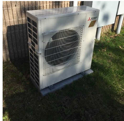
Image 11 Split-System heat pump outdoor unit
