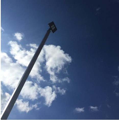
Image 3 Exterior Pole mounted LED fixture
