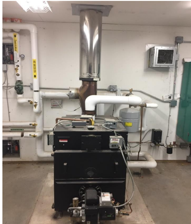
Image 5 Energy Logic Waste Oil Boiler
