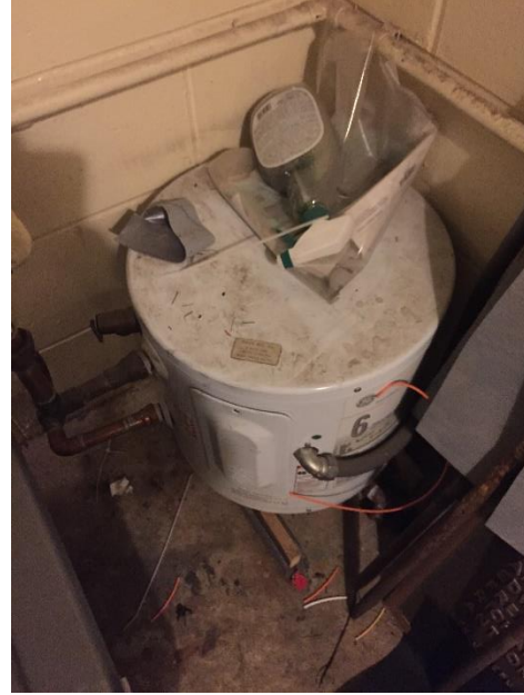
Image 13 Office Domestic Water Heater
