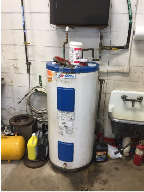
Image 12 Garage Domestic Water Heater
