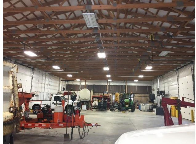
Image 4 High Bay lighting fixtures
