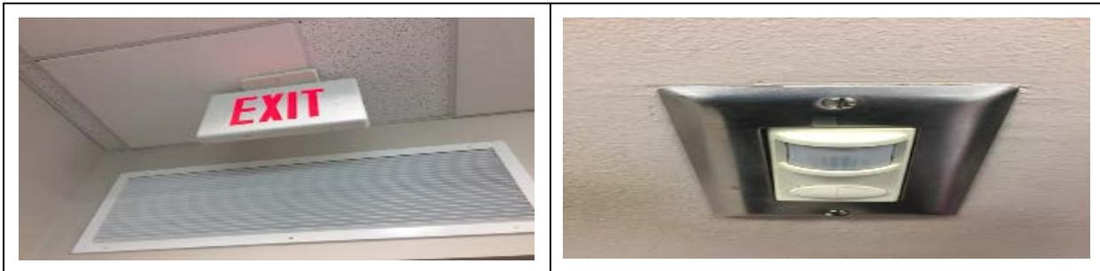
*Image 6: LED Exit Sign & Wall Mounted Occupancy Sensors*
