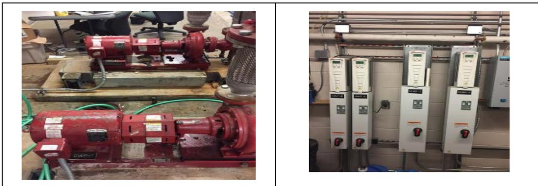
Image 9: Chilled Water Supply Pumps & VFDs
