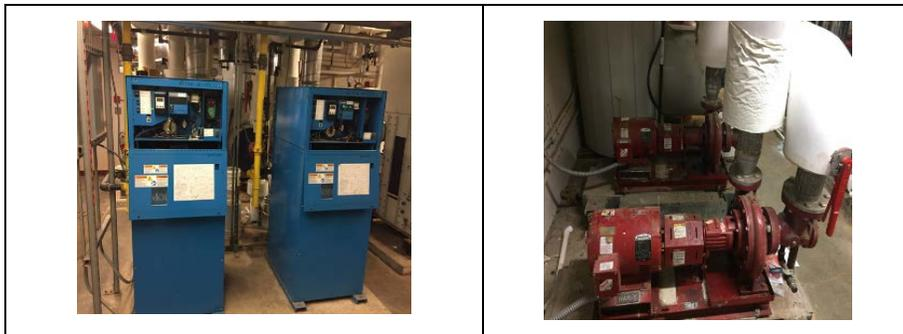
*Image 11: Heating Hot Water System*
