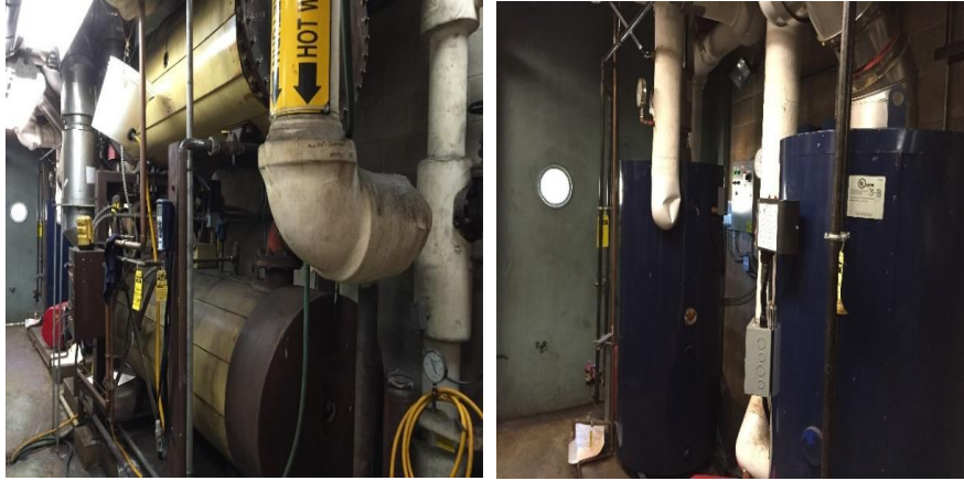
Image 4: (Left) Space Heating PVI Boilers, (Right) Seawater Heating Triad Boilers
