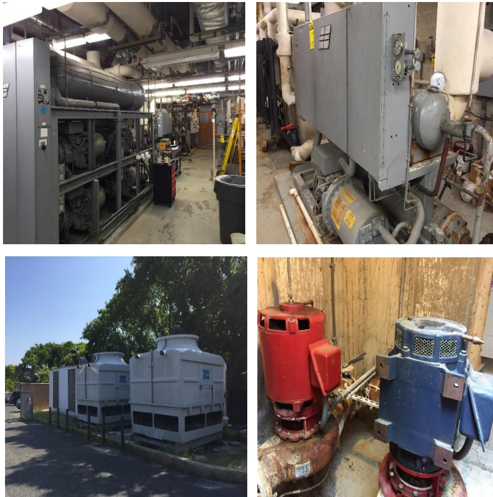
Image 3: (Clockwise) Top 2 – CH4 and CH3 located in the mechanical room, condenser water pumps, cooling tower located on the ground outside.
