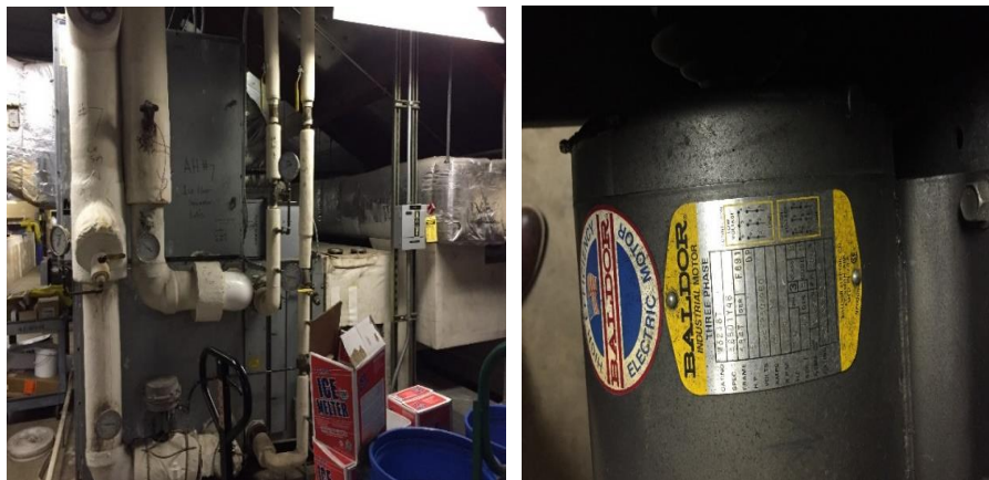
Image 5: (Left) AHU-7 located in the Penthouse, (Right) Exhaust Fan 9L Motor
