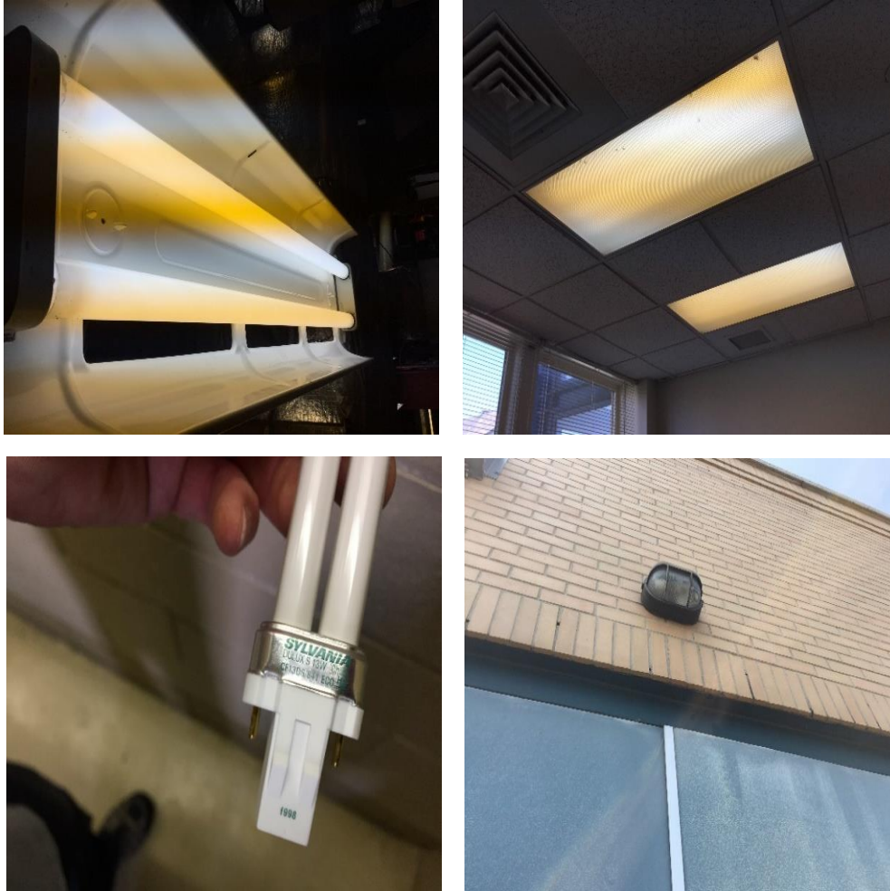
Image 2: Indoor and Outdoor Light Fixtures
