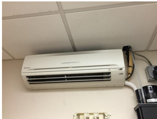
Image 3 Split AC serving IT closet
