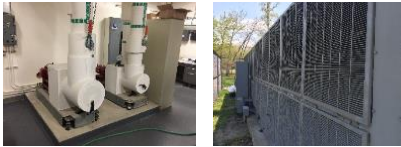
Figure 10 – Chilled Water System
