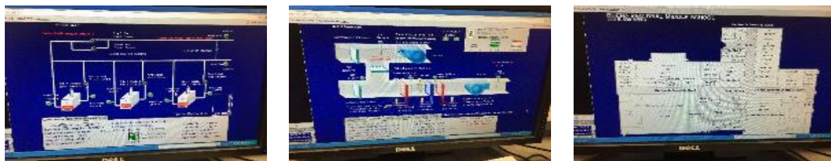
Figure 13 – Building Energy Management System Dashboards
