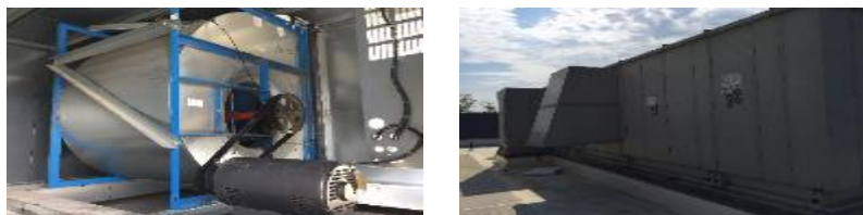
Figure 12 – Chilled Water Air Conditioning System
