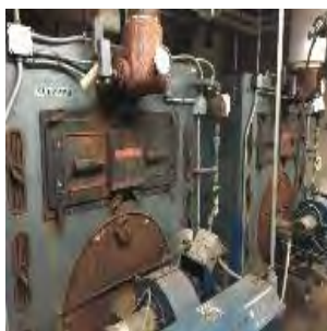
Hot Water Boilers
