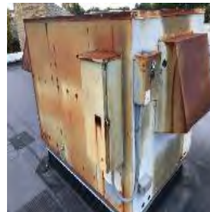
Energy Recovery Units
