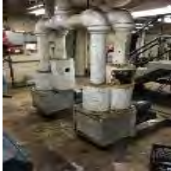
Chilled Water Pumps
