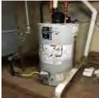
Domestic Hot Water Heater
