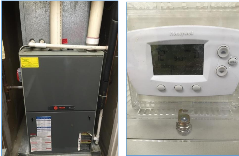
Image 5: Heating System and Thermostat
