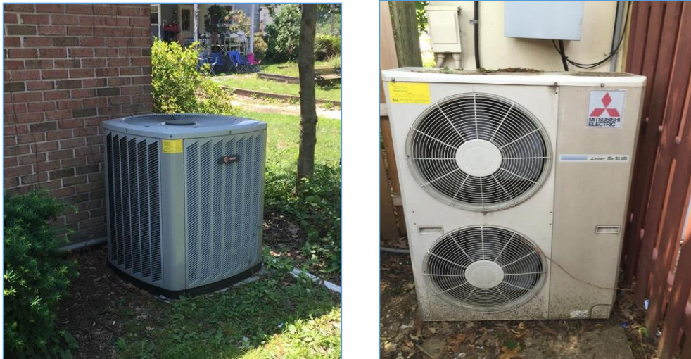
Image 6: Split System Air Conditioning Units
