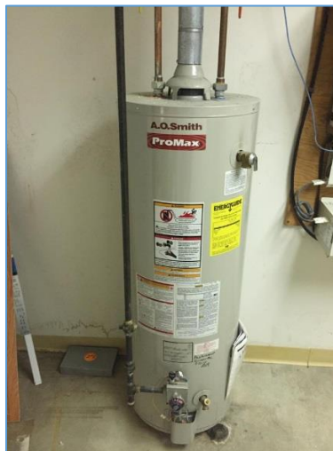
Image 4: Domestic Hot Water Heater
