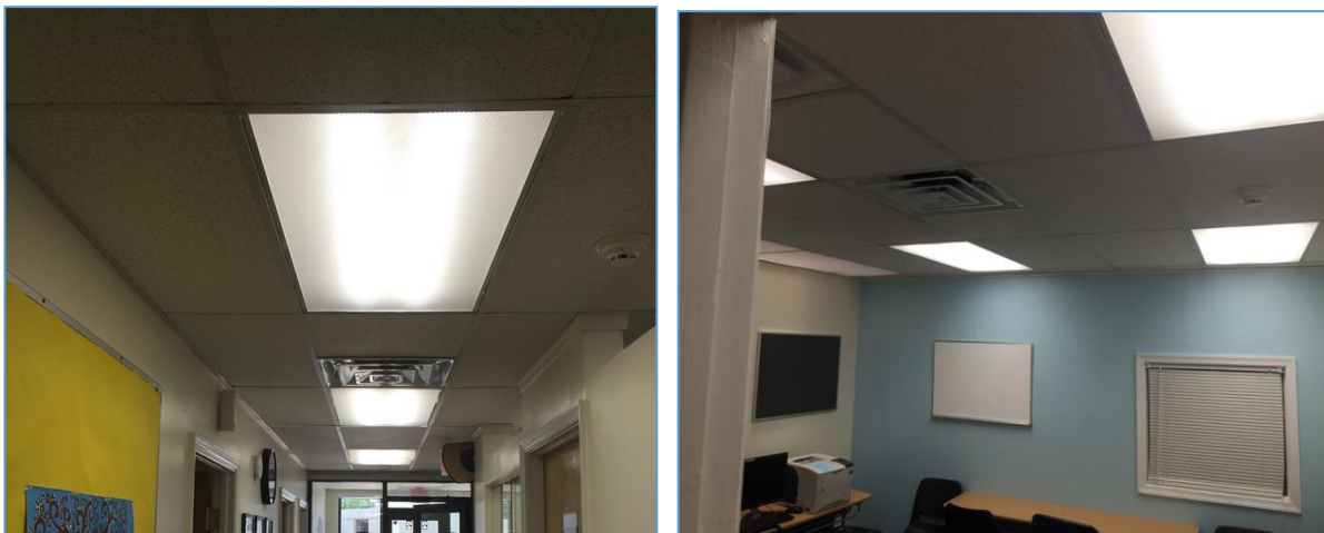
Image 3: Examples of Interior and Exterior Lighting Fixtures
