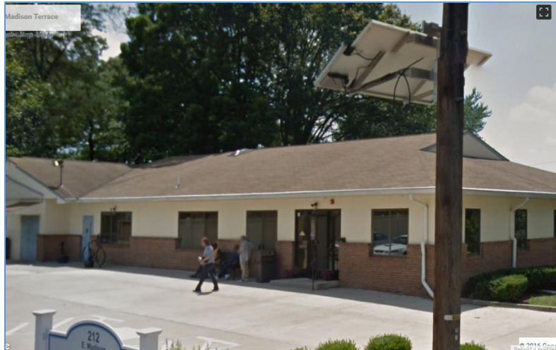
Image 9: View of Facility Showing Rooftop
