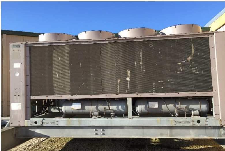
Image 4 - Chiller providing space cooling for block A
