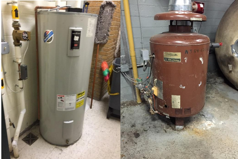
Image 6 - Domestic hot water heaters found at the facility
