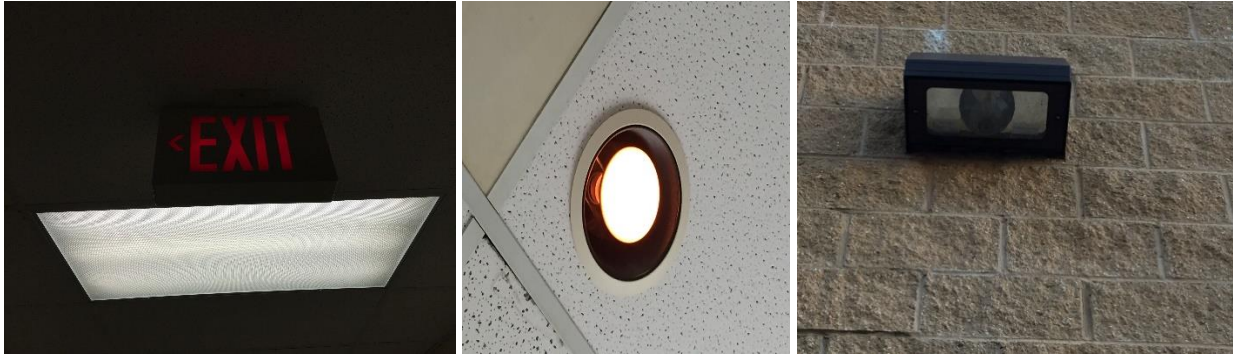
Image 2 Typical lighting fixtures at the facility
