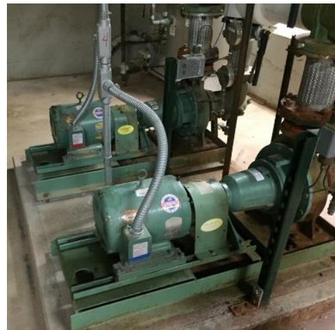
Image 3: Heating Hot Water Pumps
