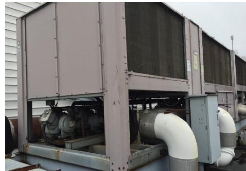
Image 2: Two Carrier 150-Ton Chillers
