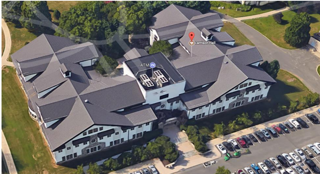
Figure 20 Rooftop Aerial View
