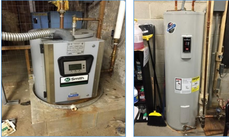
Image 4 Domestic Hot Water heaters (Left: AO Smith, Right: Bradford White)
