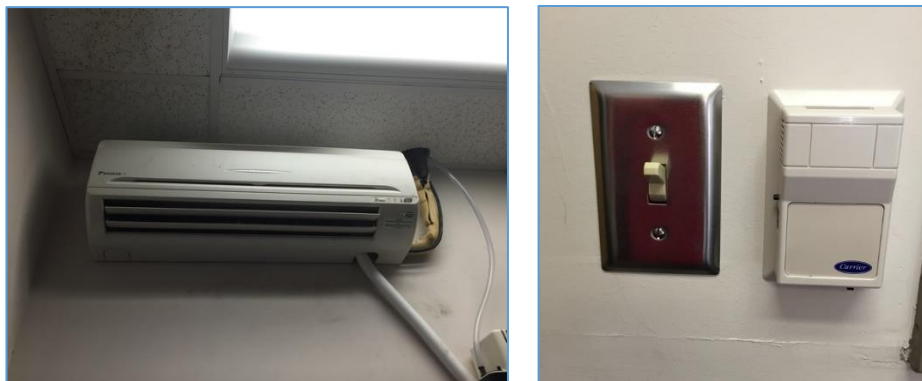
Image 3 (Left): Min-split AC unit in the server closet | (Right): Temperature controls
