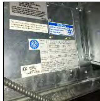
Water-Source Heat Pump
