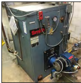
Hot Water Boiler
