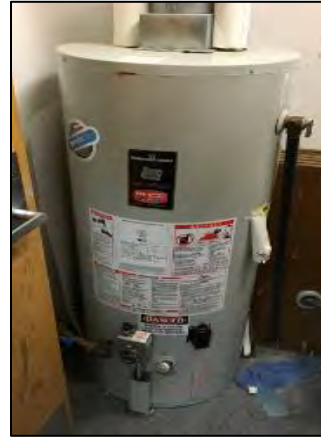
Natural Gas Water Heater
