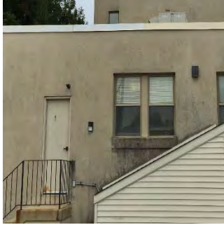
Exterior wall mounted LED fixtures
