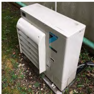
Ductless-Split system condensing unit
