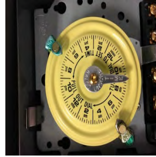
Time clock lighting control
