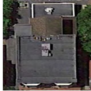
Aerial view of rooftop
