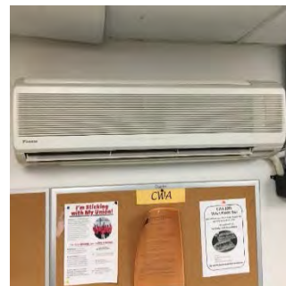
Ductless-Split system indoor unit
