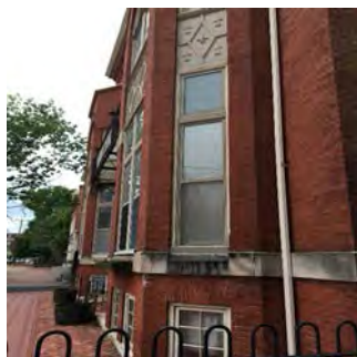
Front of building – Brick w/typical windows
