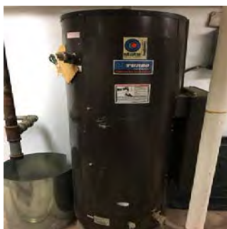
Electric domestic water heater
