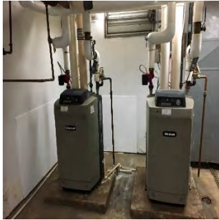
Weil – McLain hot water boilers
