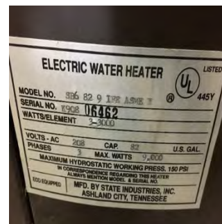
Water heater nameplate
