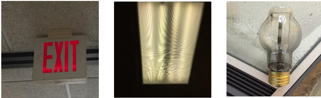
Image 1 Sample of lighting fixtures in the building
