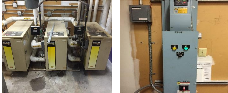
Image 2 Boiler and supply fan VFD at the boiler room
