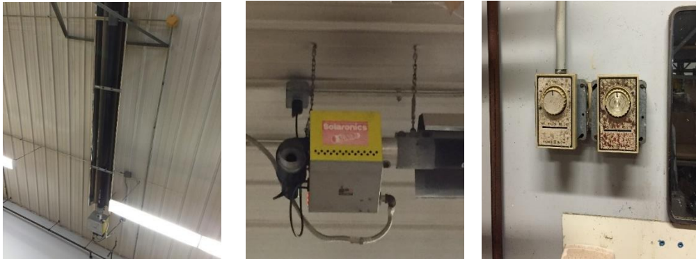
Image 4 Tube type infra-red heaters and thermostat controls
