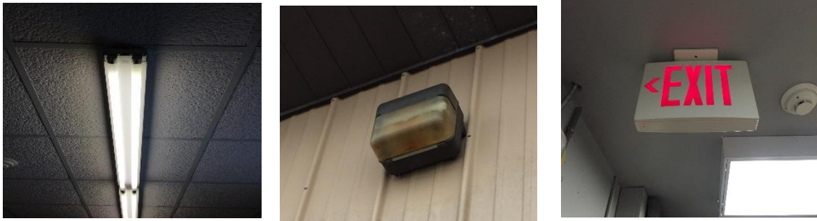
Image 2 Samples of various lighting fixtures
