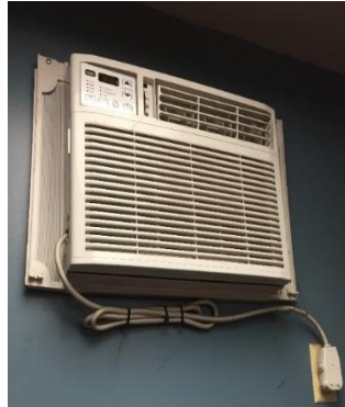
Image 3 Window AC providing space cooling
