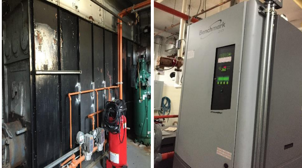
Image 3 Hot water systems at the school
