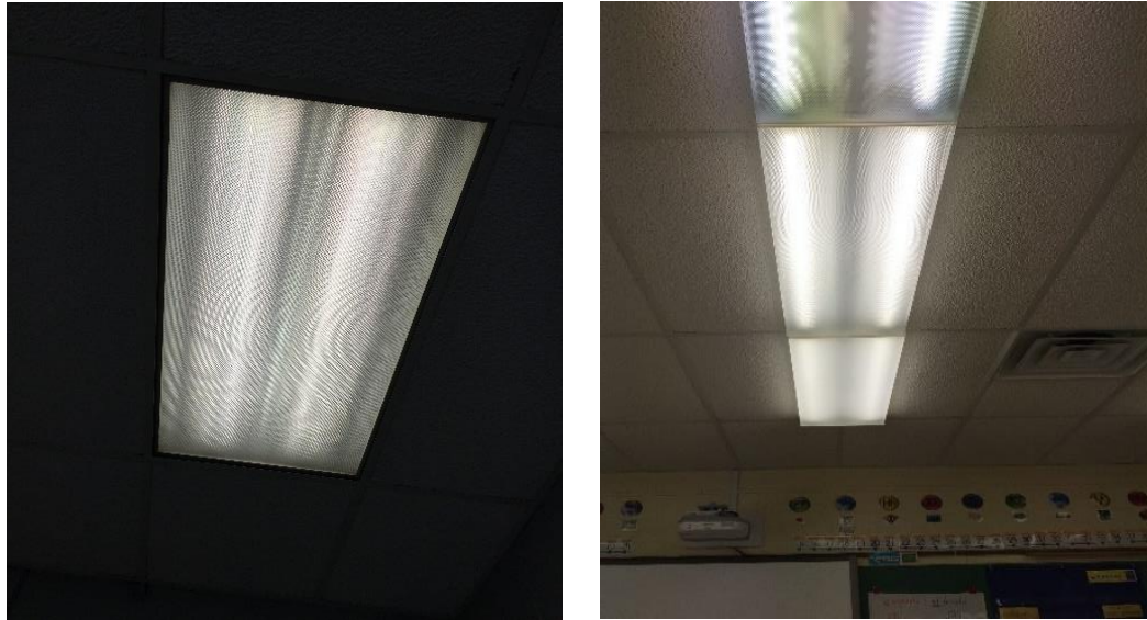
Image 2 Typical lighting fixtures at the facility
