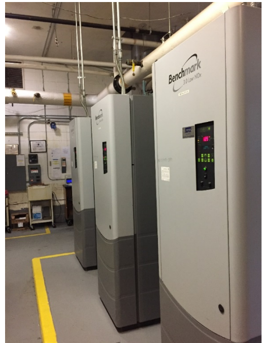
Condensing Boilers
