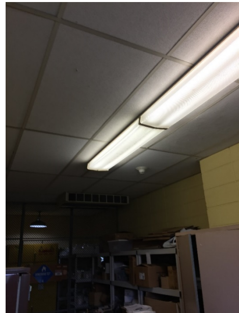
Typical Lighting Fixture
