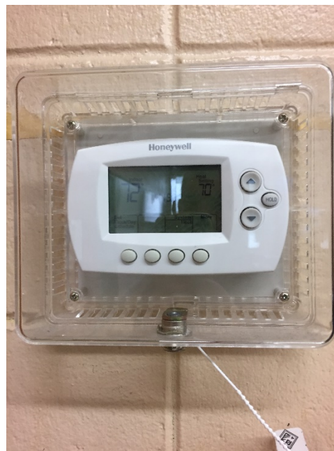
Typical Control (HVAC)
