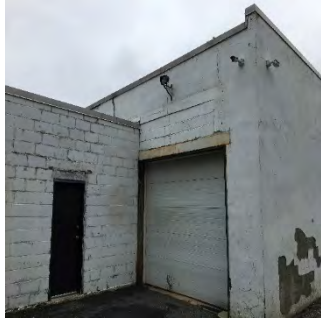
Typical exterior doors and walls
