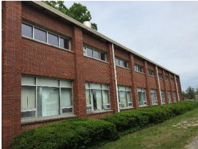
Figure 7 - Building Exterior and Envelope
