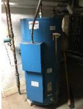
Figure 12 – Domestic Hot Water Heating Equipment
