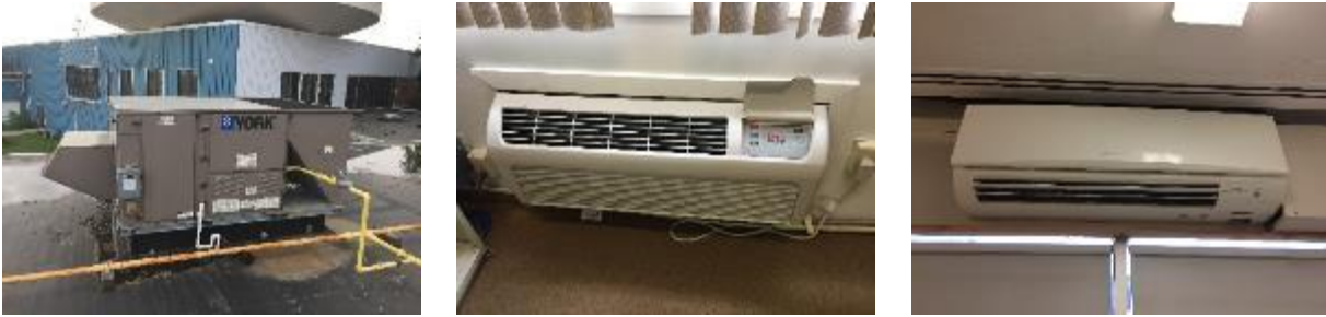
Figure 10 – Direct Expansion Air Conditioning Equipment
