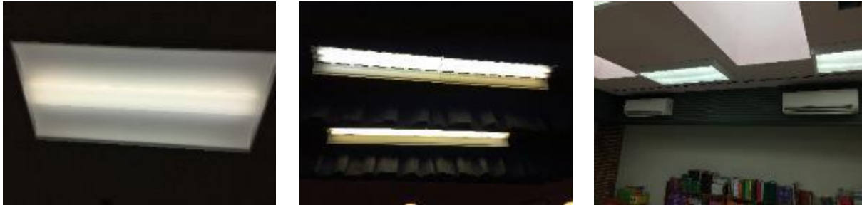
Figure 8 – Lighting System Fixtures
