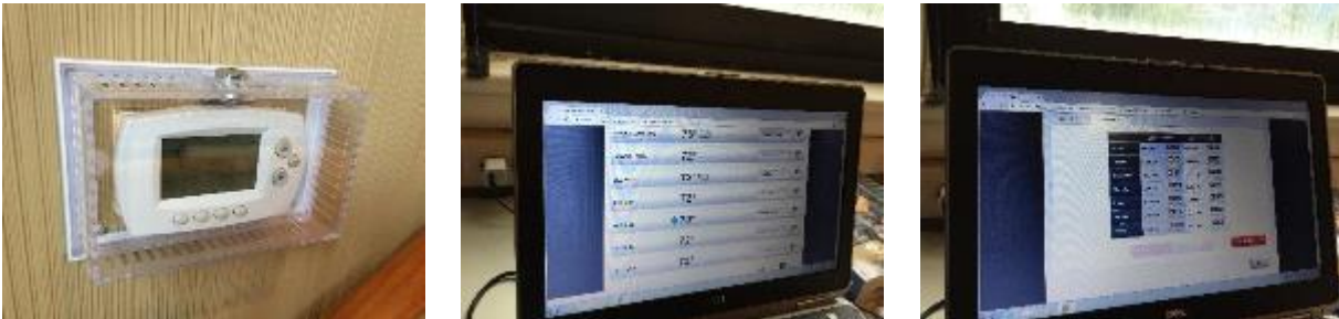
Figure 11 – Building Energy Management System Settings
