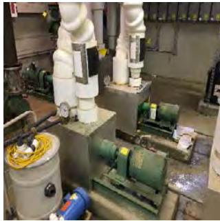
Chilled Water Pumps
