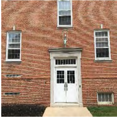
Building Exterior Wall Lights
