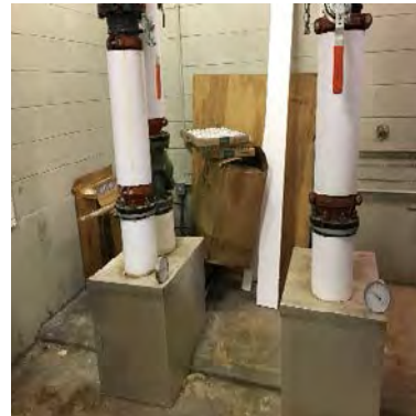
Hot Water Pumps
