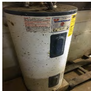
Domestic Hot Water Heater
