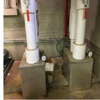
Chilled Water Pumps
