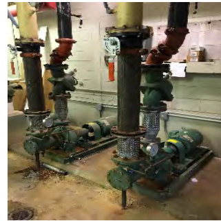
Condenser Water Pumps
