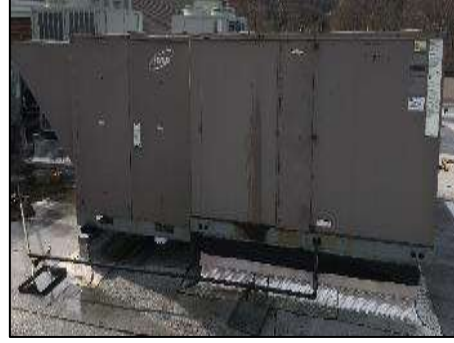
Cafeteria Packaged Unit
