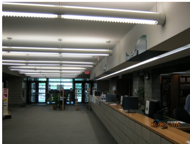
Figure 7- Lighting Fixtures at the Library
