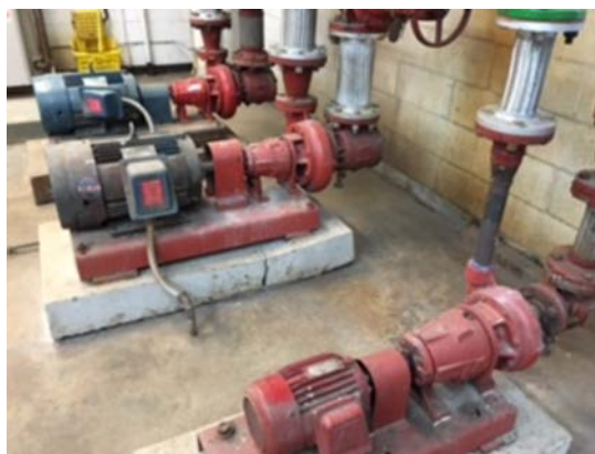
Figure 9 - Chilled Water Pumps
