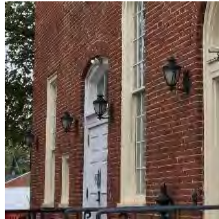
Image 7. Exterior Wall Pack Fixtures
