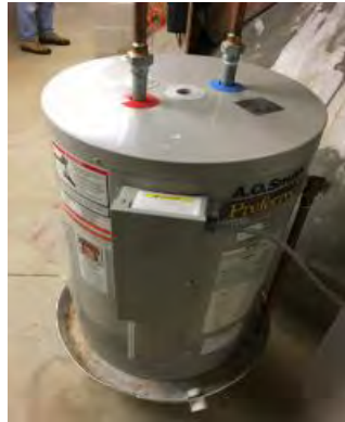
Image 10. Electric Water Heater
