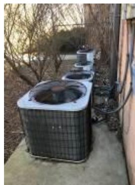
Four Carrier split system AC units of various capacities and efficiencies
