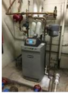
Weil McLain Ultra 230 CT boiler
