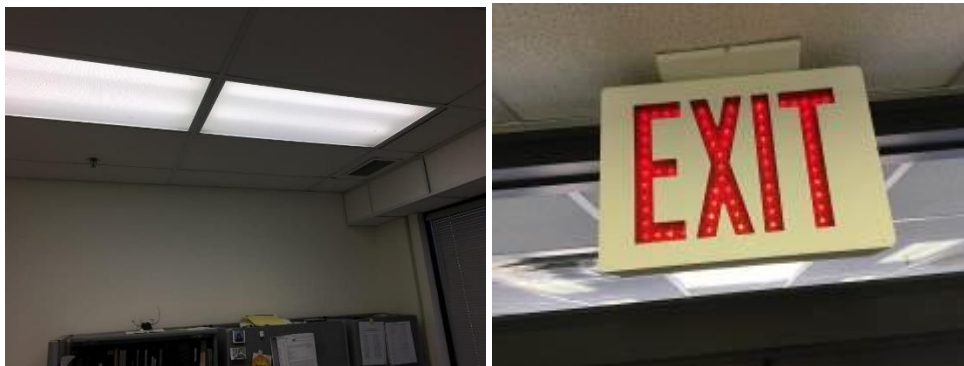
Office Area lighting consists of T8 fixtures. There are LED exit signs throughout
