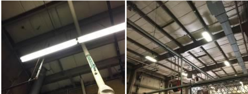
Garage Bay Lighting consists of T8 and T5HO fixtures
