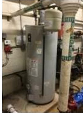
Bradford White gas fired hot water heater
