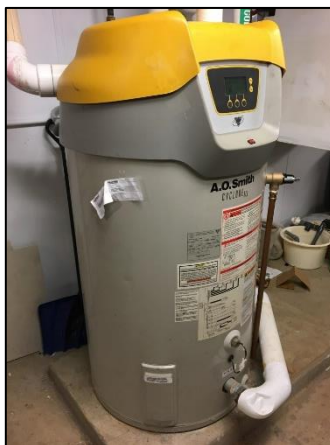
A.O. Smith gas fired hot water heater
