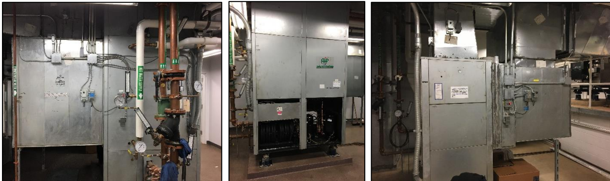
Heat pump units AC2, AC3, and AC5
