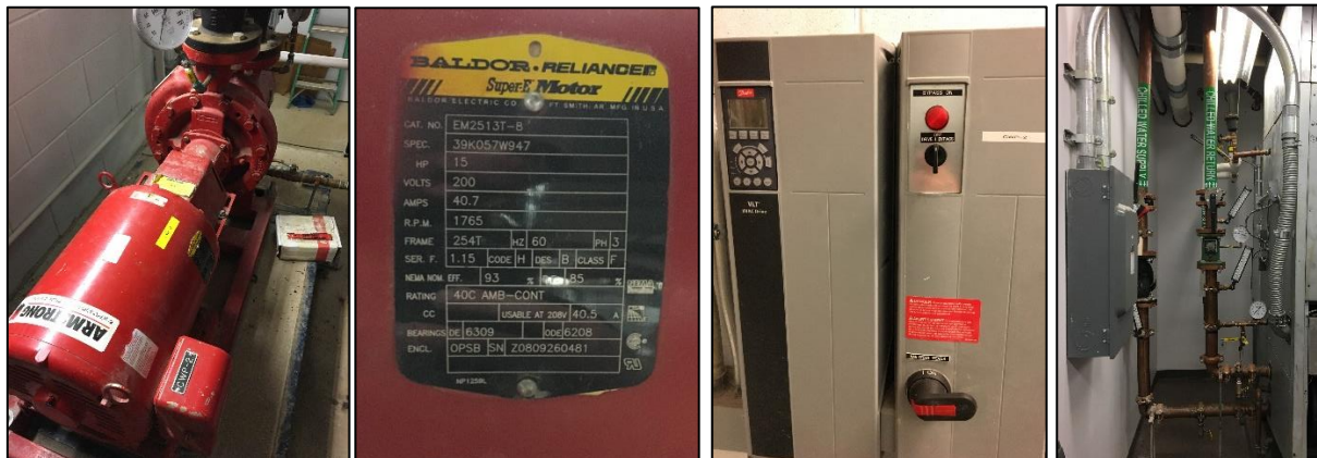
Chilled water pump, low-voltage drive, and ACI
