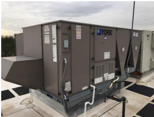
Direct-expansion (DX) packaged AC units
