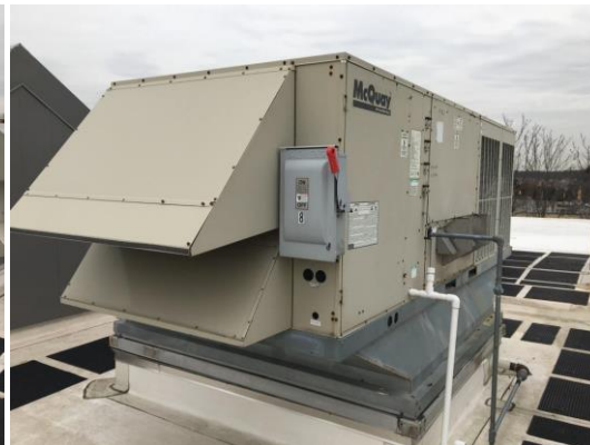
Direct-expansion (DX) packaged AC units
