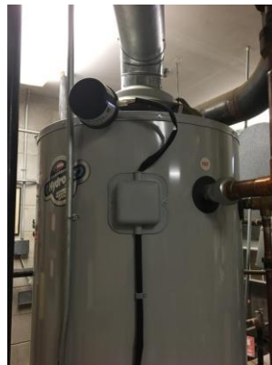
Bradford White gas fired hot water heater
