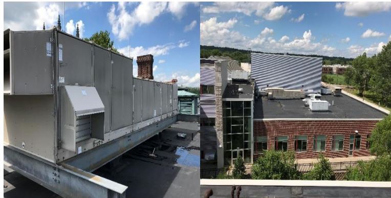
Image 7 AHUs on Roof
