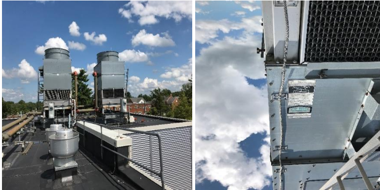
Image 5 Cooling Towers on Roof
