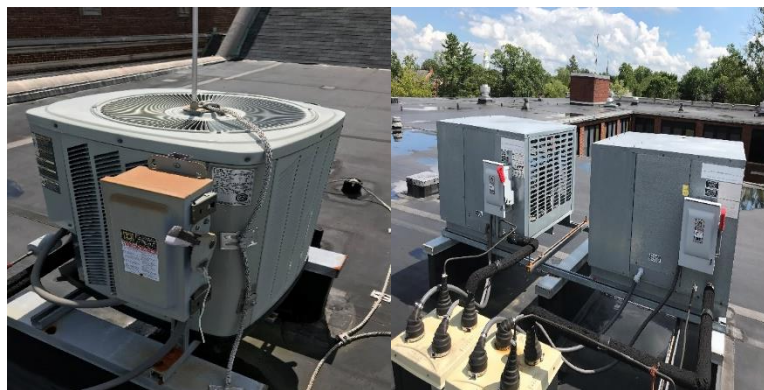
Image 8 DX Units on Roof
