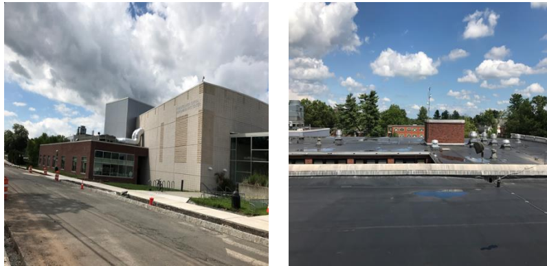
Image 1 Building Exterior and Roof
