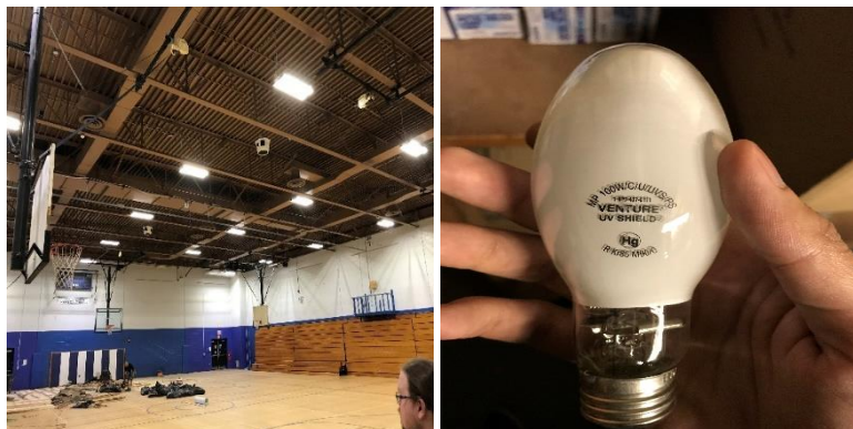
Image 2 Lighting Fixtures in Gym and sample bulb
