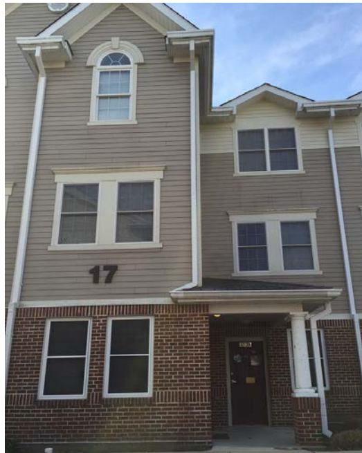
Image 1: Townhouse Windows and Doors
