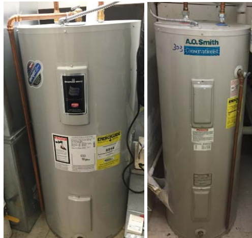
Image 7: Domestic Hot Water Heaters
