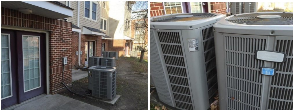
Image 4: Split System Condenser Units behind Each Townhouse
