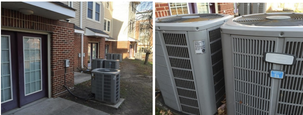
Image 4: Split System Condenser Units behind Each Townhouse
