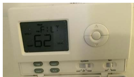
Image 5: Programmable Thermostats in Each Townhouse
