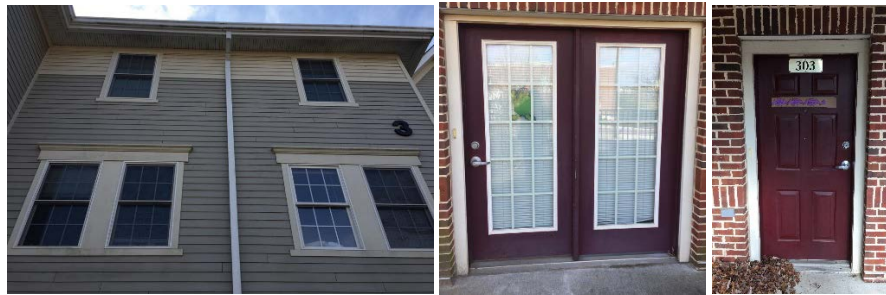
Image 2 (cont.): Townhouse Windows and Doors
