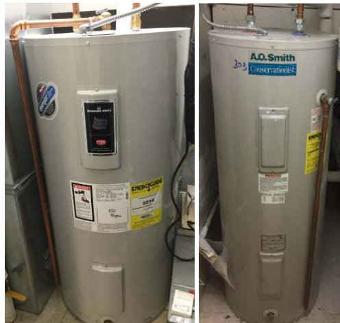
Image 7: Domestic Hot Water Heaters
