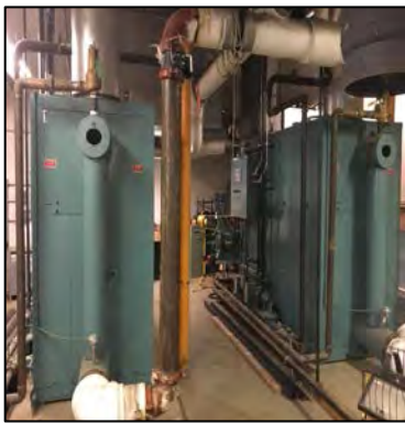
Heating Hot Water Boilers
