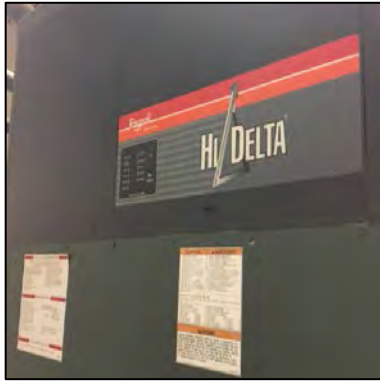
Domestic Hot Water Equipment
