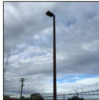
Exterior Lighting Fixtures
