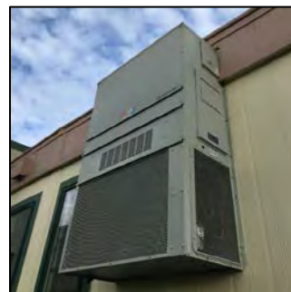
Through-The Wall Air Conditioner
