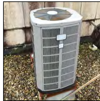
Split System Air Conditioner Condenser
