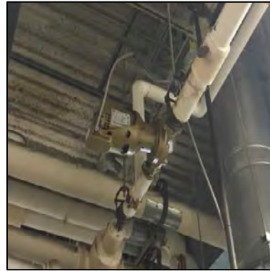
DHW Distribution Pumps
