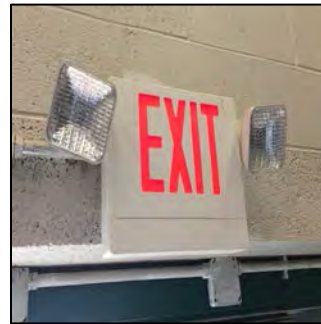
LED Exit Signs
