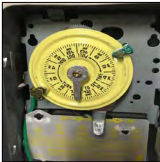
Exterior Lighting Timer Control
