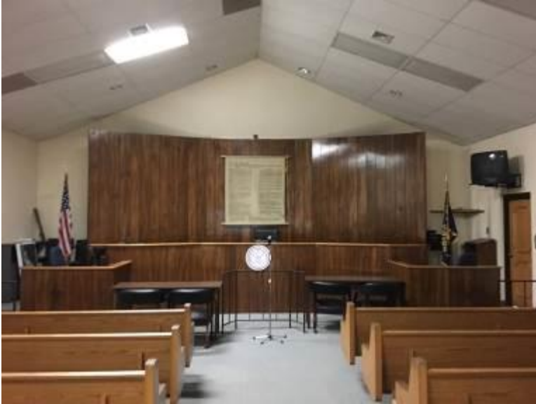
Image 3 – T8 Fluorescent Lighting (court room)
