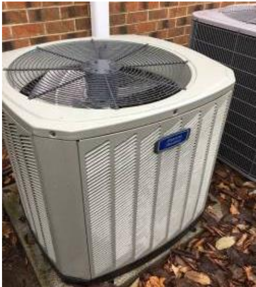
Image 5 – Split-System AC (condenser)
