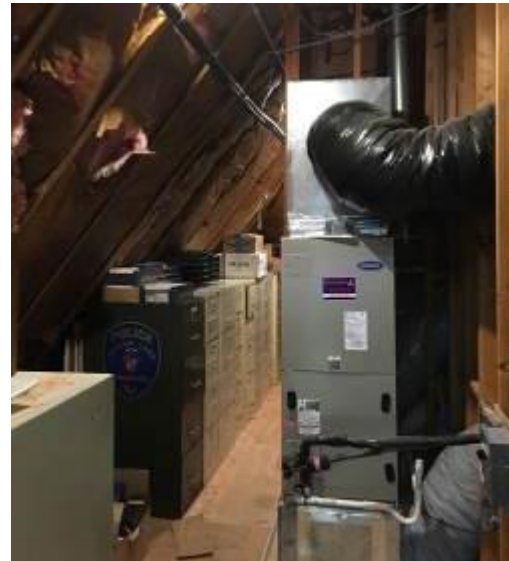
Image 6 – Split-System AC (supply fan/evaporator)
