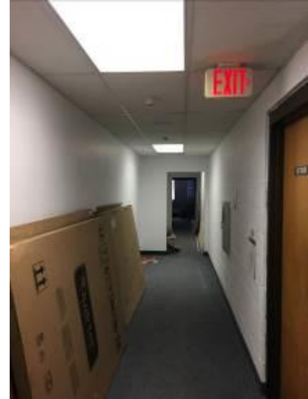
Image 4 – T8 Fluorescent Lighting (hallway)
