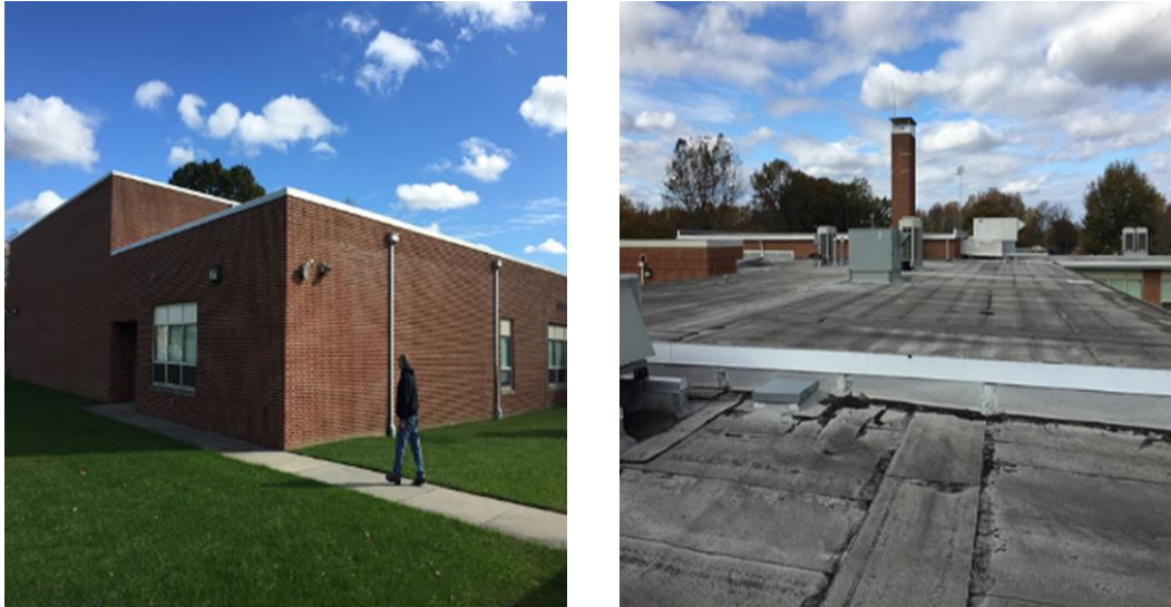
Image 1: Building Wall & Roof
