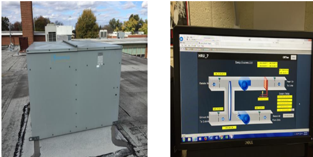
Image 5: Energy Recovery Ventilation System
