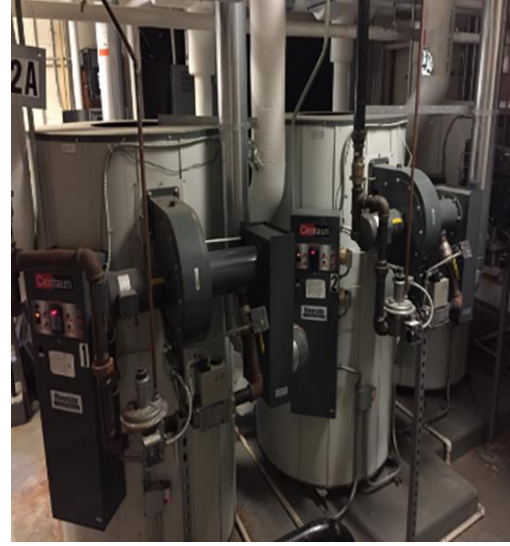
Image 3: Heating Hot Water System
